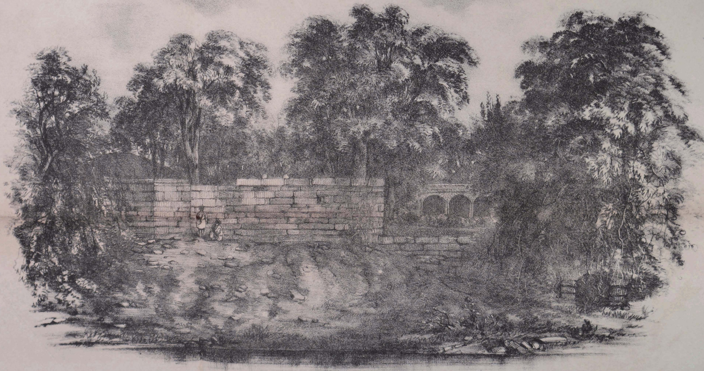
WEST BANK OF KUND SHEWING RETAINING WALL.
